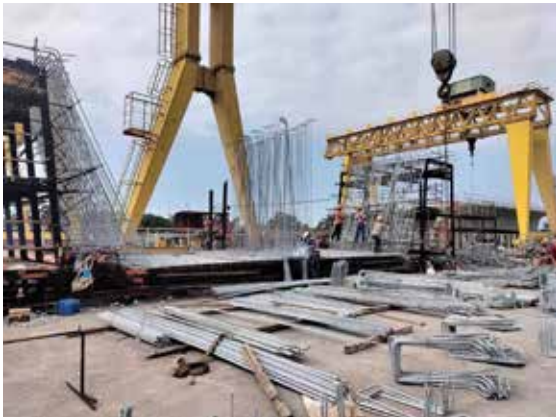
(a) 底板及腹板鋼筋綁紮
