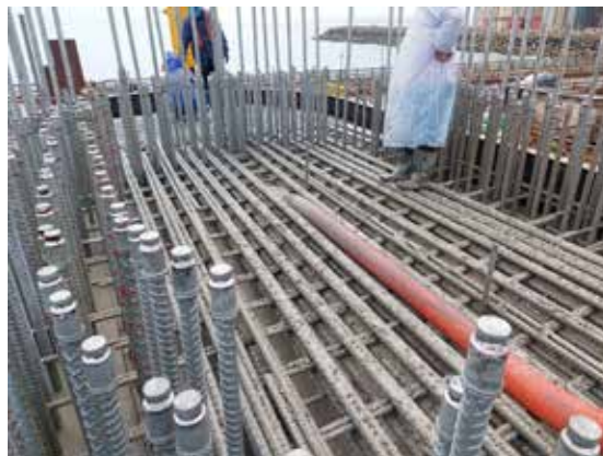
(c) 橋柱鋼筋續接器鍍鋅
