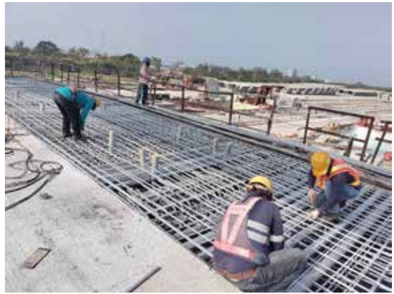
(b) 頂板鋼筋綁紮
